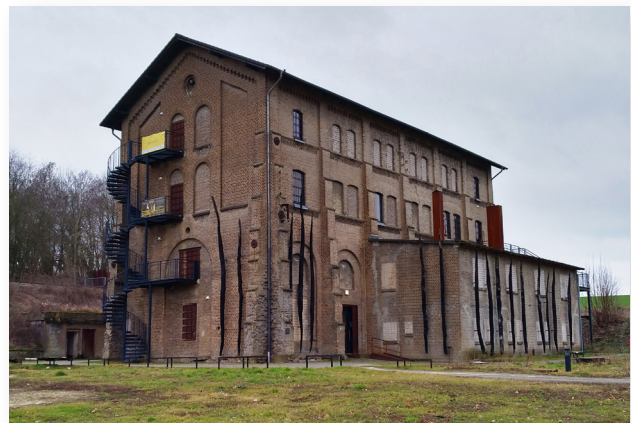
Abb. 19: Pumpstation des Augustaschachts Ohrbeck (Foto: N9713, CC BY-SA 4.0 < https://creativecommons.org/licenses/by-sa/4.0/ >, via Wikimedia Commons)
